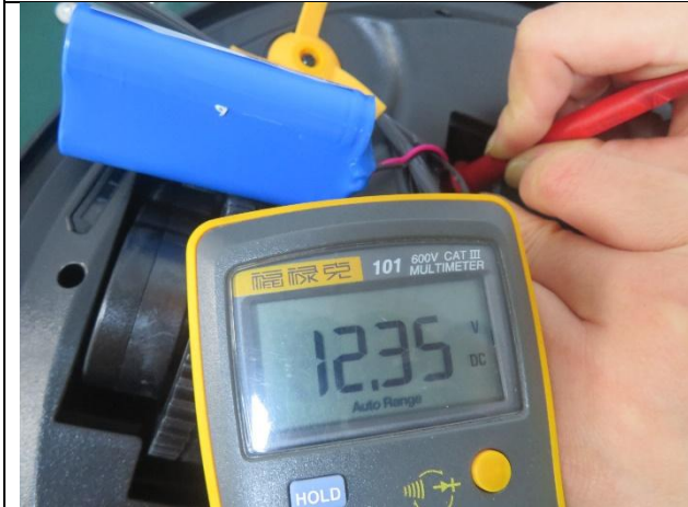
159. Battery voltage measurement
